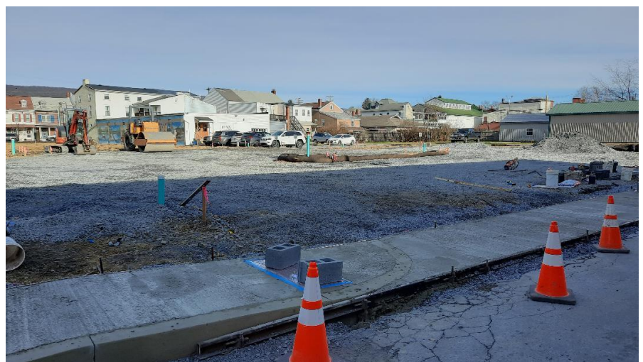
Construction at the State Street Square lot
